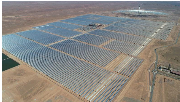
Figure 1 Utility-scale solar plants [SolarReviews].
