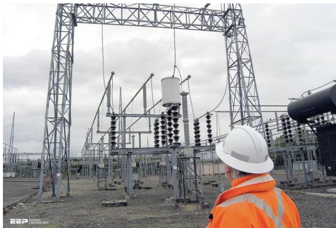
Figure 1 Substation construction [electrical-engineering-portal].
