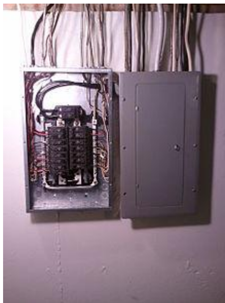
Figure 1 Distribution board
