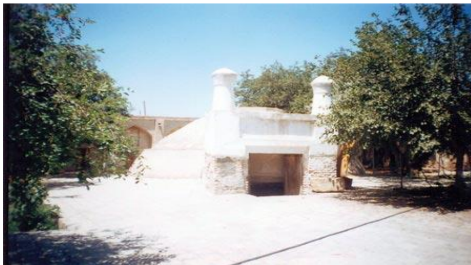
Picture 2. Semi-underground Sardoba has a caravanserai.
