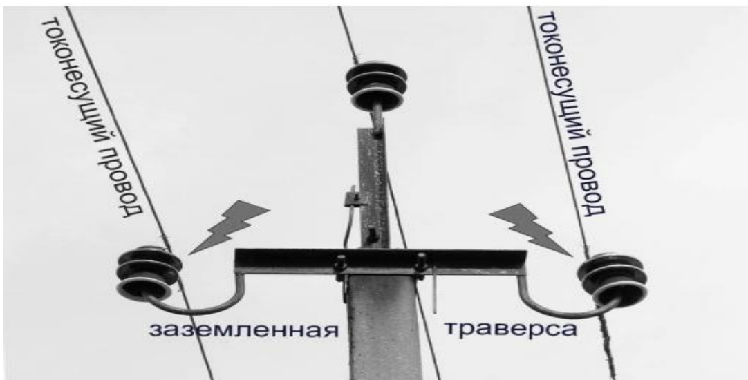
Fig. 2 the small distance between the current-carrying and grounded elements in the area of the head of the support of the 6-10 kV overhead line determines the high danger of the structure for objects of the animal world.
