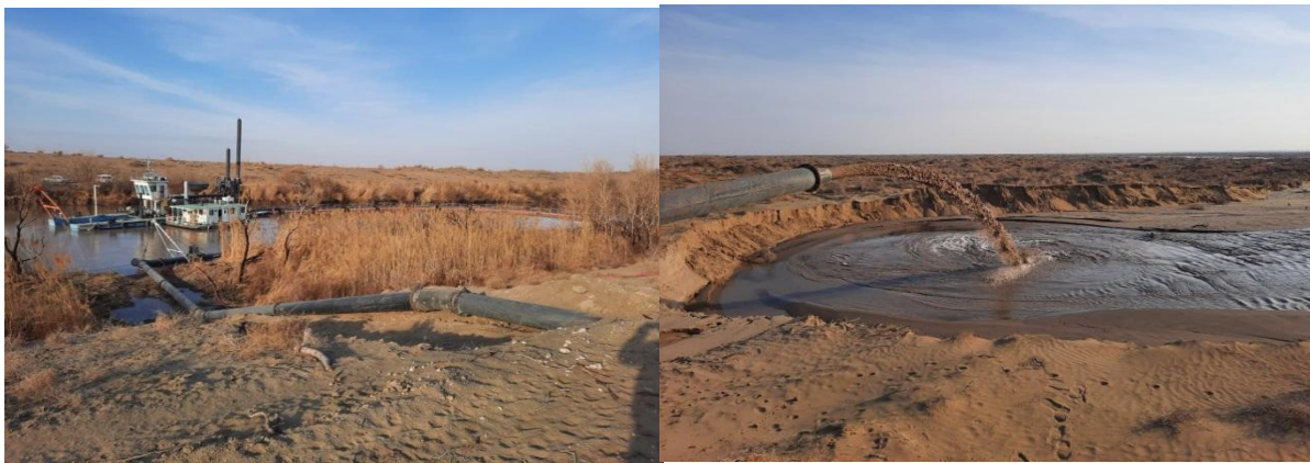
Fig. 1-Dredger in the ABK-1 channel
