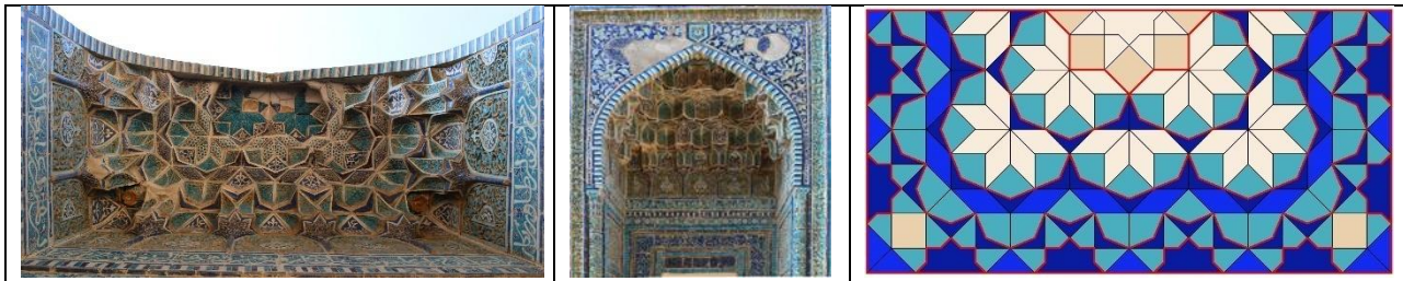
Fig.2 Architecture details of muqarnas Shodi Mulk Oko Mausoleum at the Shah-i-Zinda, Samarkand, Uzbekistan. Photo and geometric analysis of Shakhboz Mustafiev.
